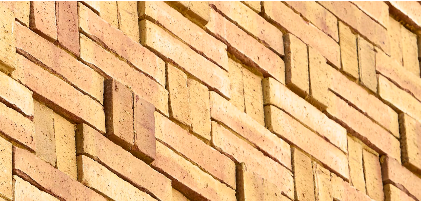
Flemish bond of double stretchers and headers
