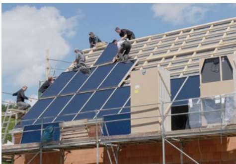
Assembly of the solar thermal and photovoltaic modules on the south-facing roof surface: the solar system that was integrated into the roof surface allows the combination of solar heat, photovoltaics and roof windows.
